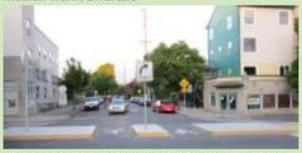
Median traffic diverters restrict through motor vehicle movement while providing a refuge for bicyclists to cross the busier roadway in two stages.
